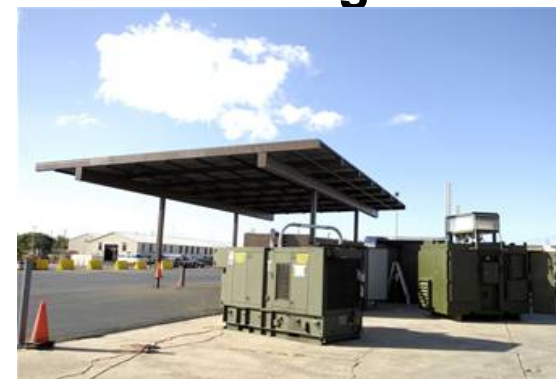
Hydrogen fuel station - Hickam
