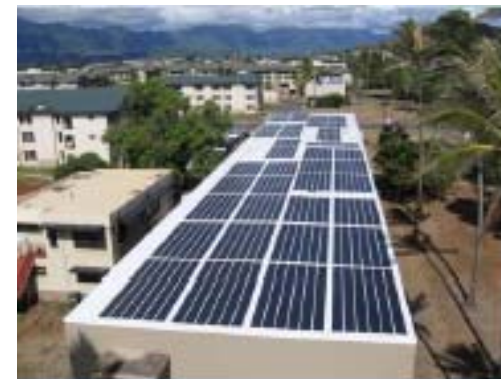
Rooftop PV K-Bay
